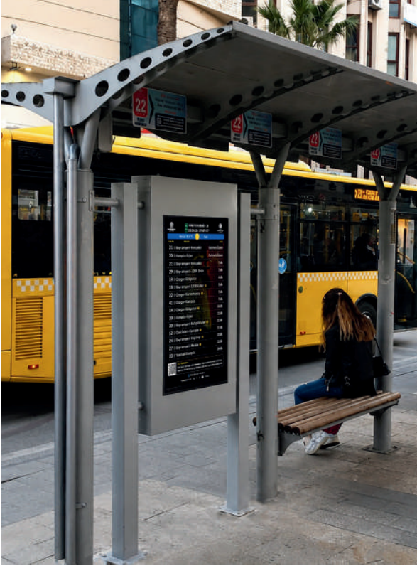
Derince Municipality – Smart Bus Stop Display
